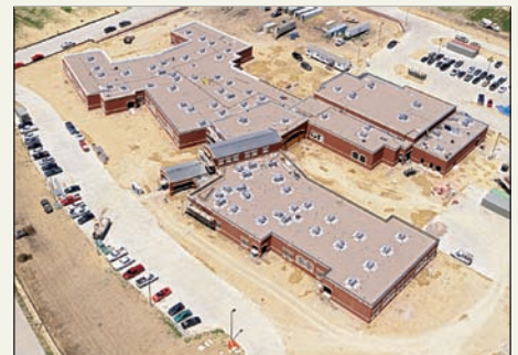
SENDERA RANCH EAST ELEMENTARY SCHOOL - HASLET, TX
