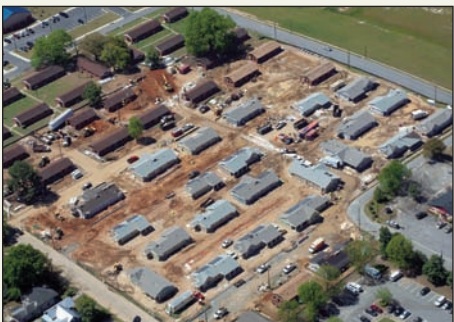
FELTON HOMES APARTMENTS - MACON, GA
