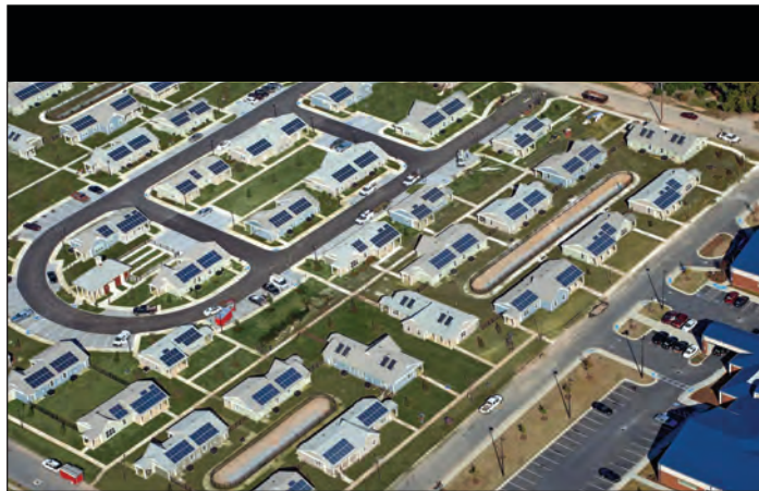
McShane Construction led the transformation of the 1940's era Felton Homes Apartments in Macon, Georgia into one of the largest multi-family solar projects in the country to date, offering solar generated energy for each of the 50 duplex homes redeveloped within the complex.
