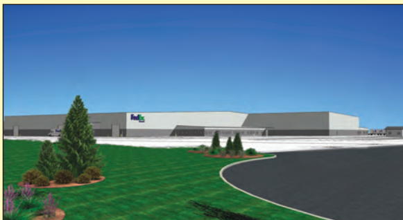
SunCap Property Group selected the design/build team of McShane Construction and Ware Malcomb to provide comprehensive design/build construction services for a new 221,619 square foot FedEx Ground facility in Windsor, Connecticut, that includes 99 truck docks and six drive-in doors.
