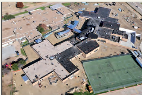
MEMORIAL ELEMENTARY SCHOOL – PLANO, TX
