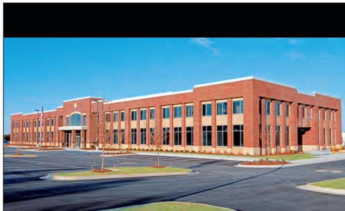
On behalf of developer, Triad Properties Corporation, McShane Construction's Auburn office recently completed the new 62,500 square foot, two-story office and training center in Huntsville, Alabama for the General Services Administration tenant, Defense Acquisition University.
